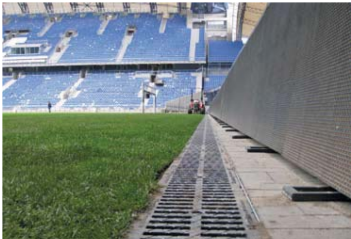
EURO 2012 stadium in Poznan EM-Stadion in Posen
